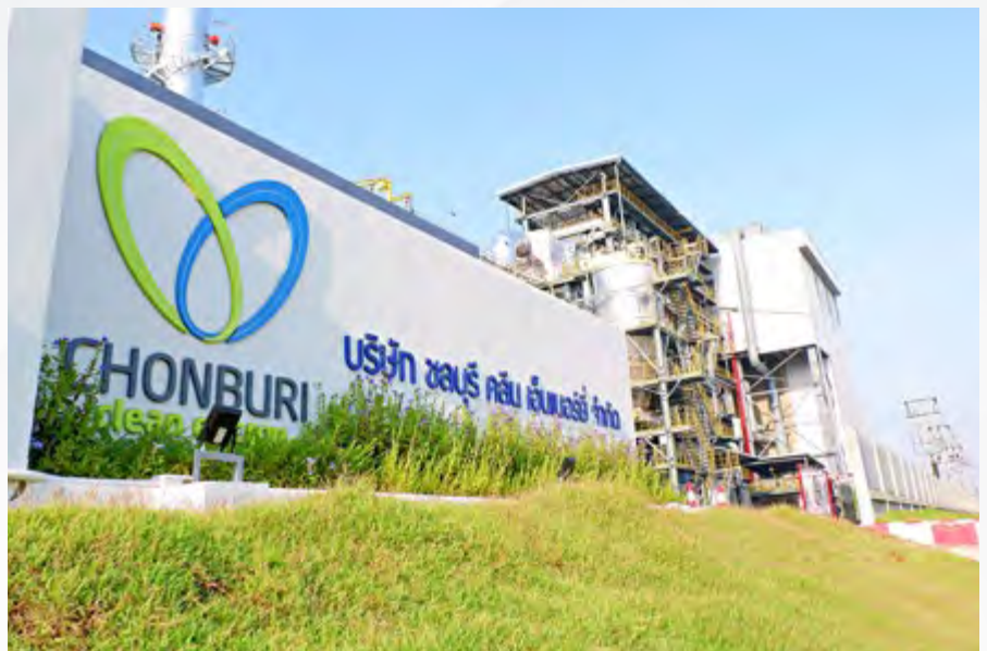
Chonburi Clean Energy (Thailand) benefits from this risk-based Smart O&M approach
